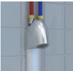
Exposed water inlets
